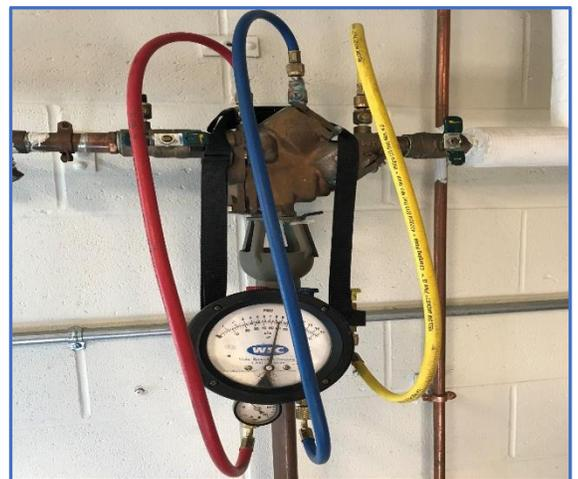
water, the backflow test will then ensure that the device is in a failed state. The inspector will allow a certain time period to have the device repaired or replaced. Most devices on the market have repair kits available.
